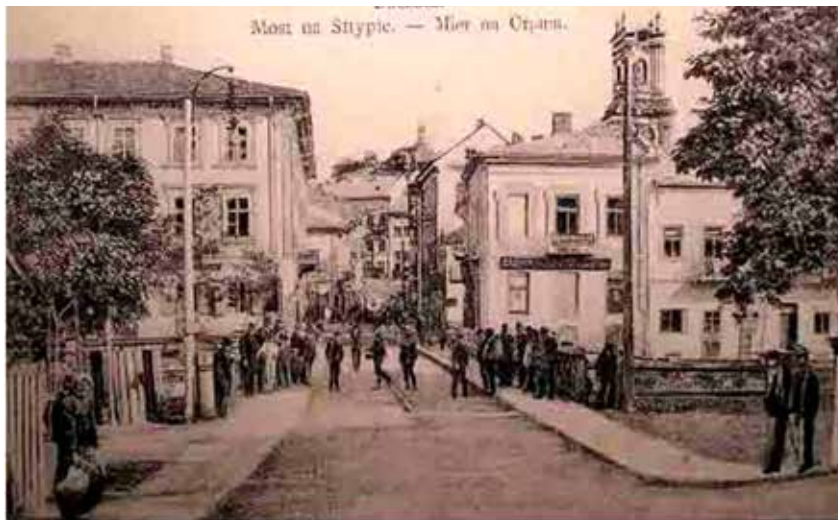
Buchach Bridge over the river Most.
