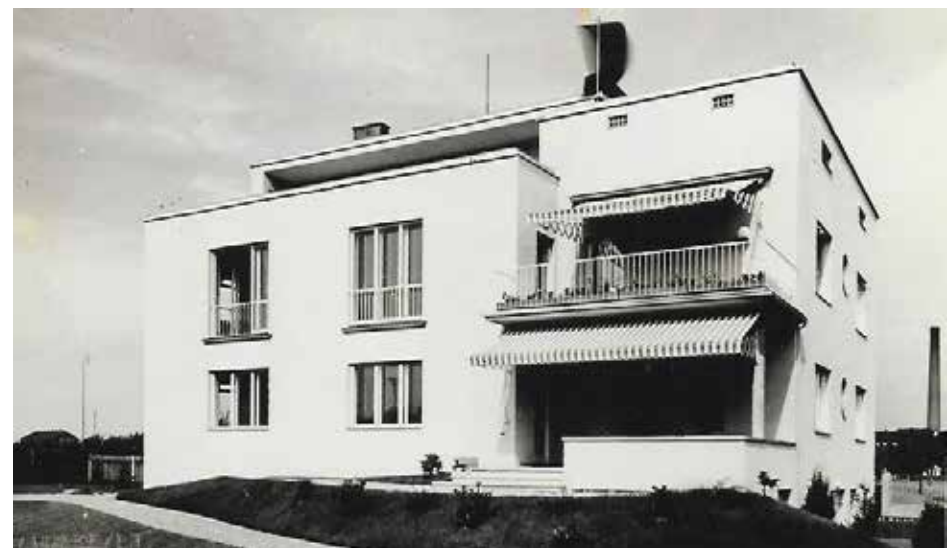
Wellnerova 21, Olomouc. This three level villa was designed by architect Jaques Groak for Siegfried Briess and built in 1937.
